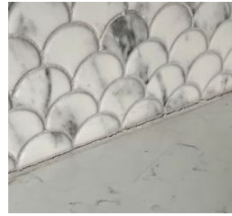
Grout Crack
