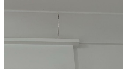
Caulking Crack
