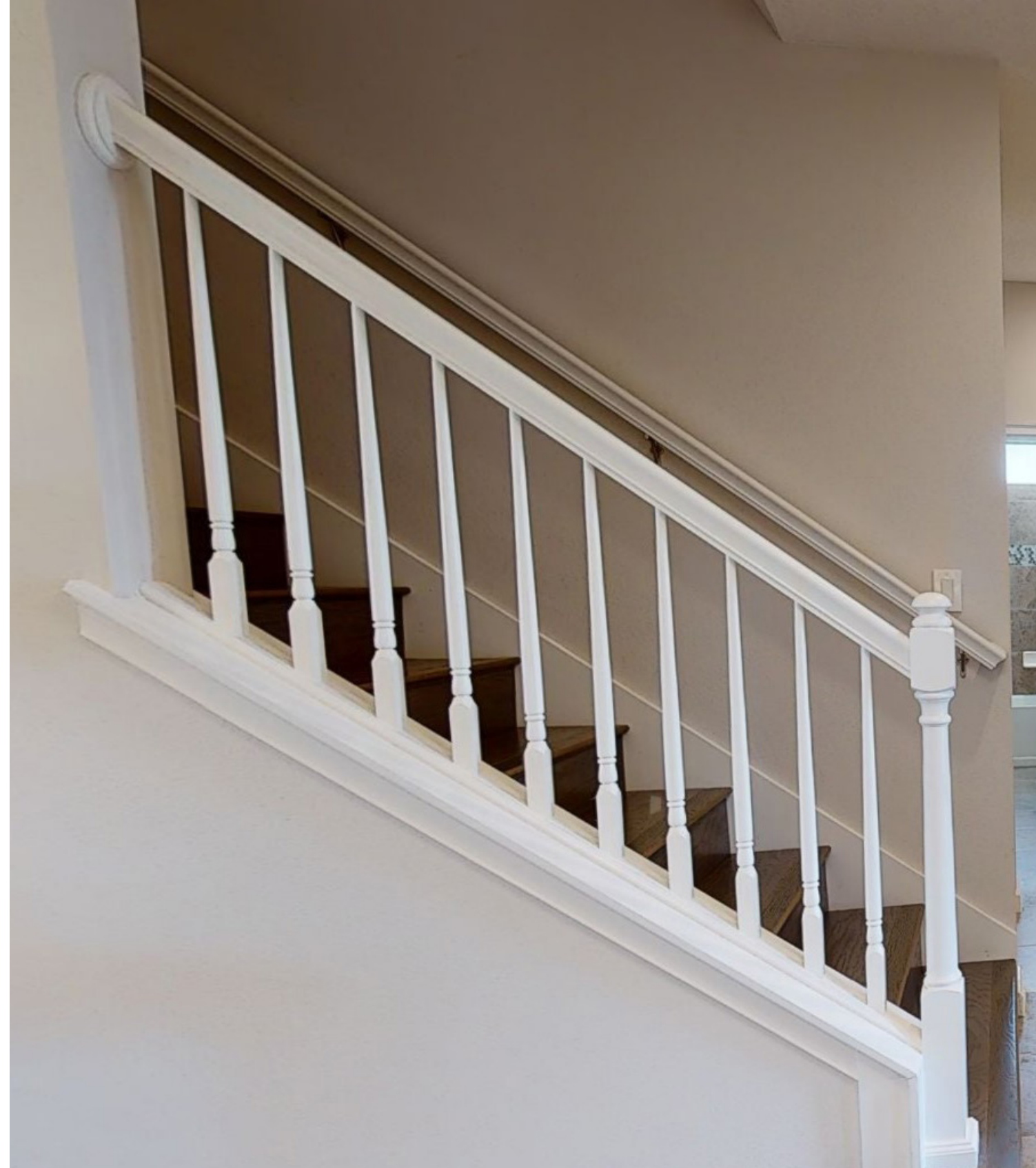
Painted Wood Railing
