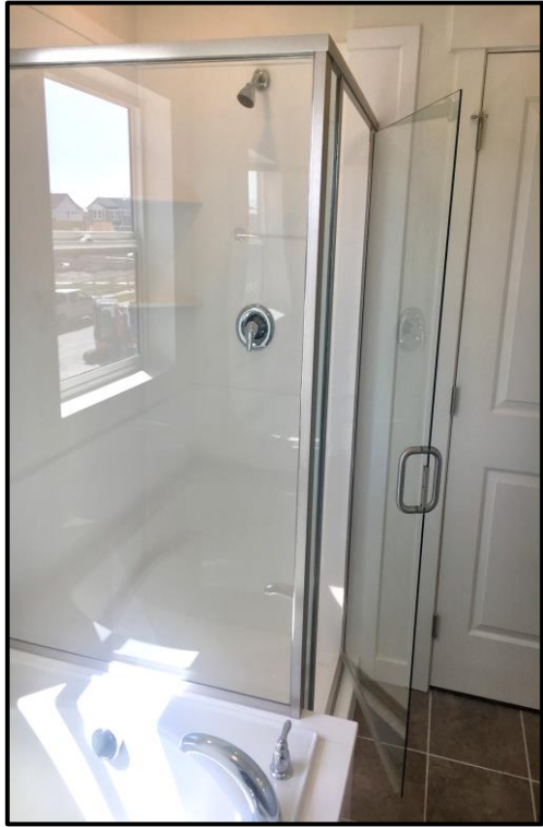
Shower Door is Upgraded to Frameless 1/4" Thick Glass 70" Tall
