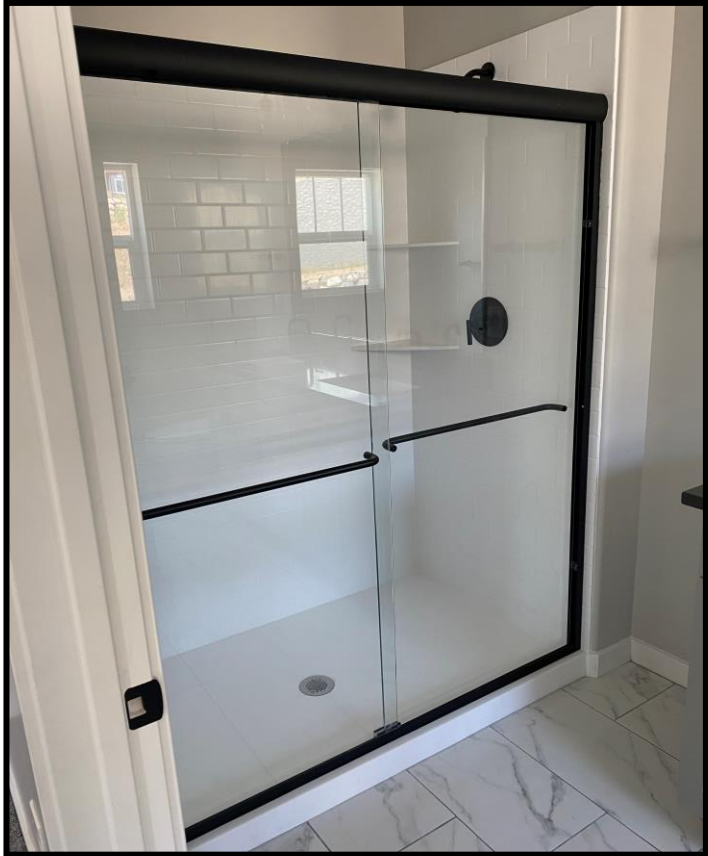
Shower Door is Upgraded to Frameless 1/4" Thick Glass 70" Tall
