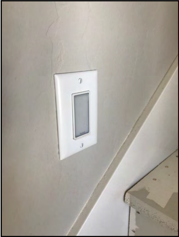
LED Stairway Lighting
