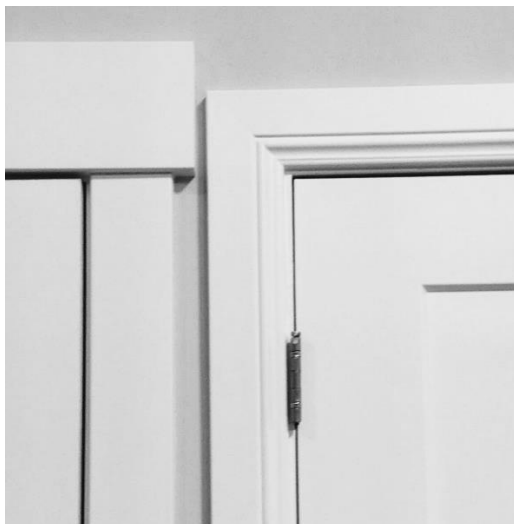
Small baseboards/door casing
